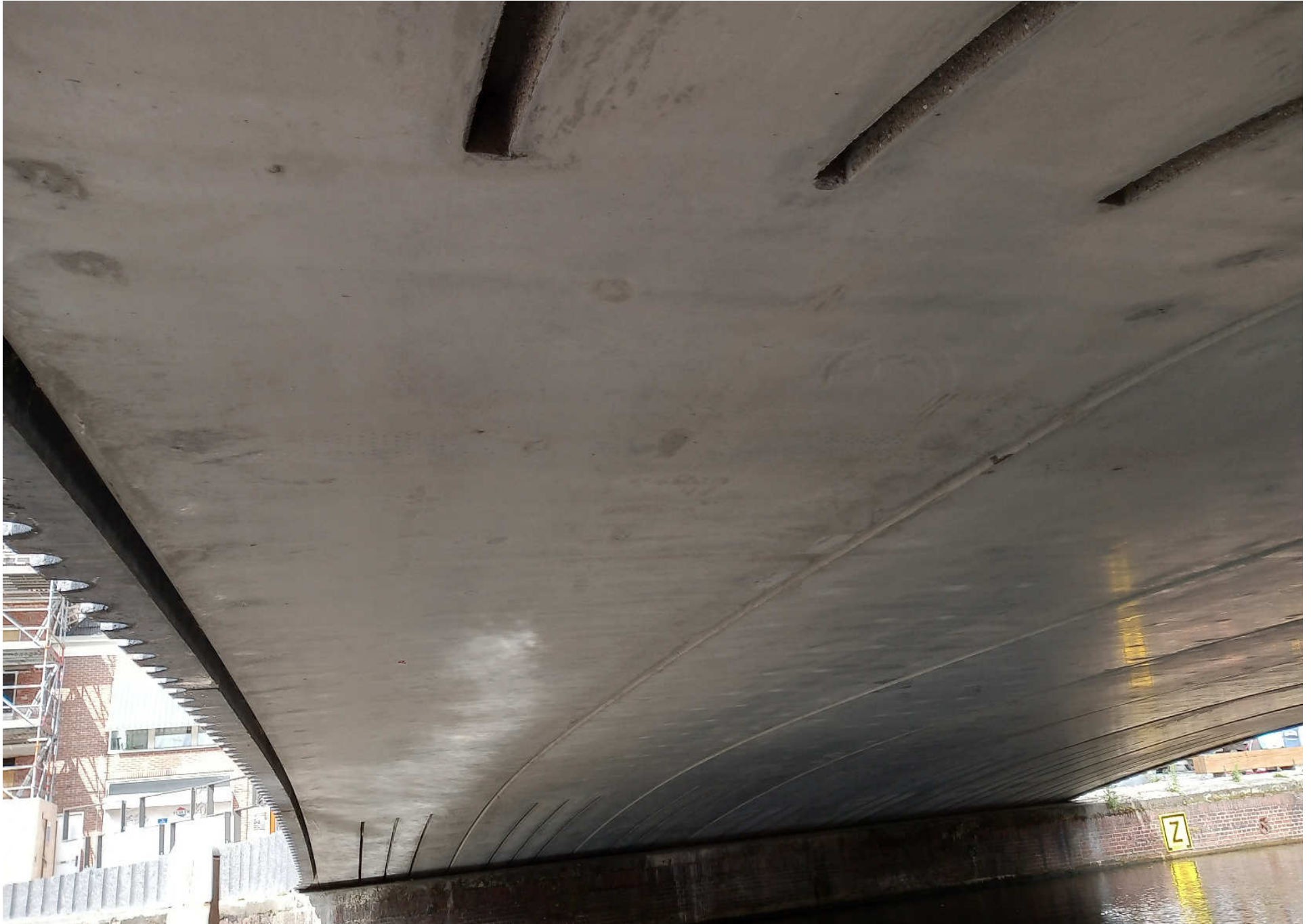
Scratches for bads under the bridge deck, Kattenbrug, KorthTielens architecten, DS
